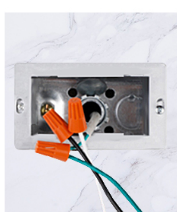
STEP2 Connect the wire with the connector
