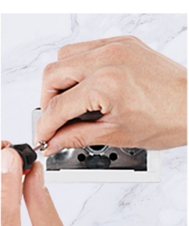
STEP1 Iron sheet installed in the junction box
